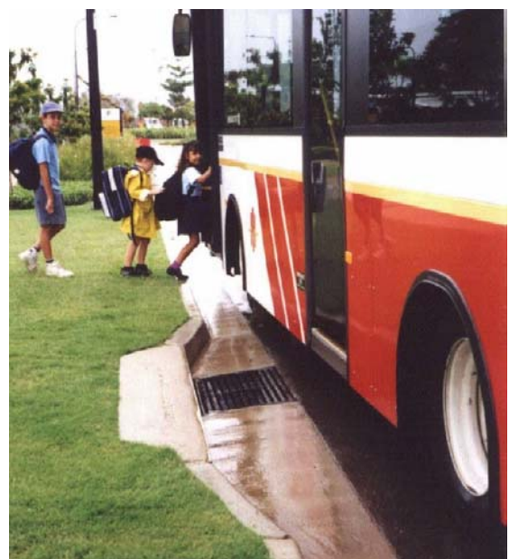
Manning lip-in-line Inlet - 210mm kerb setback
