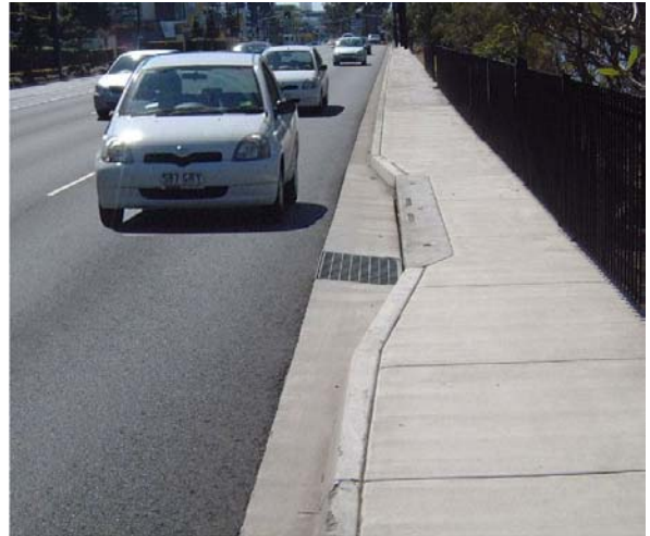
Trafficability is compromised by set back kerb
