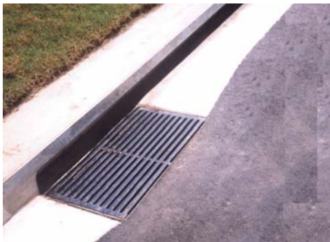
Manning Kerb-in-line Inlet
