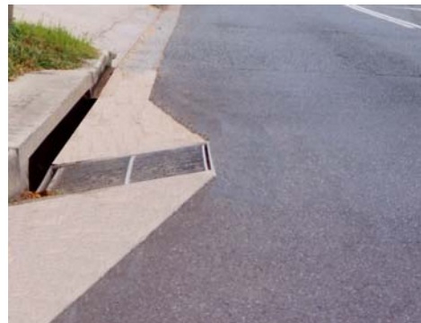
BCC Type A Kerb-in-line Inlet
