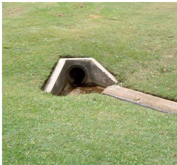
4. Mountable kerb directing flow to pipe entrance
