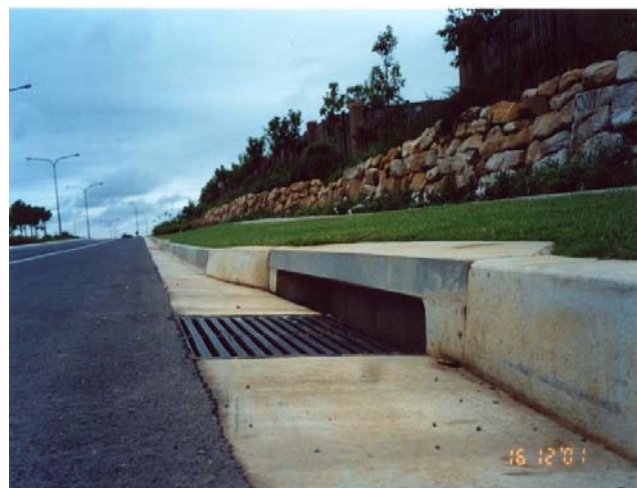
3. Manning grate with 100mm kerb inlet
