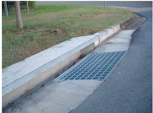
1. A child may pass through or be wedged in a 125mm high kerb opening
